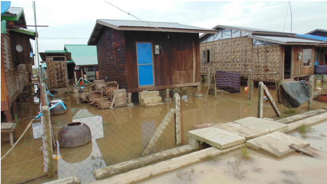
Photo 1 – Flooding in the housing lot.
