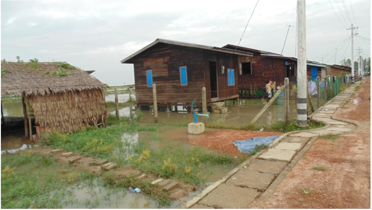
Photo 4 – Flooding around a water pump.
